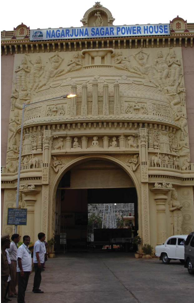
14. Façade of Nagarjunasagar Power Station.
