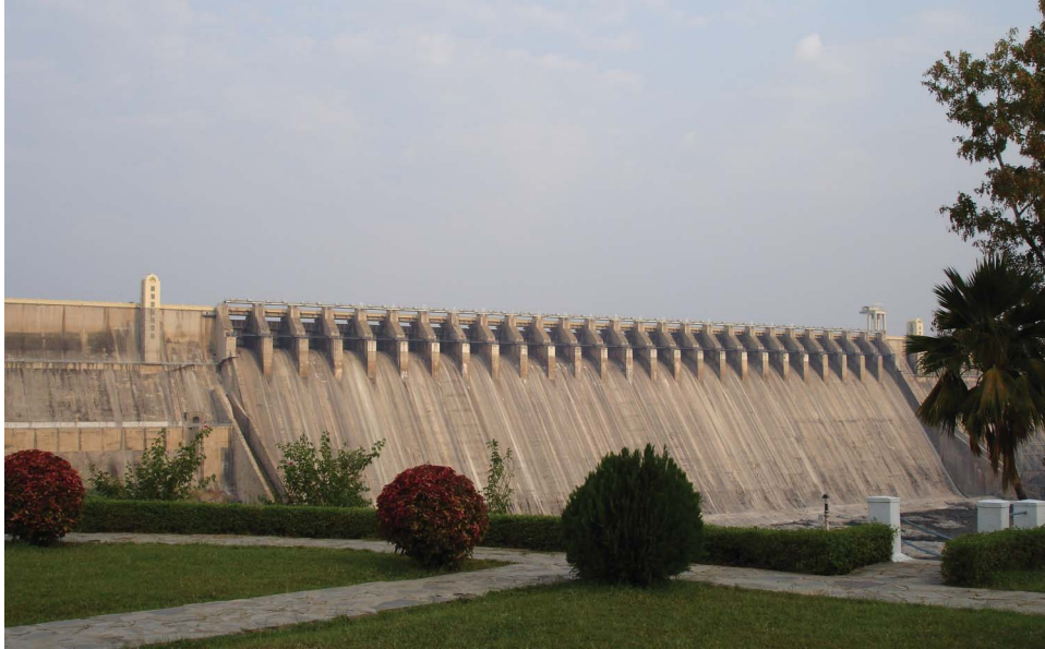
6. The Nagarjunasagar dam.
